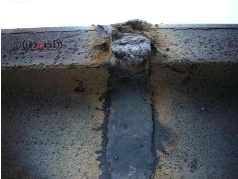
Last layers surfaced with hard wire.
