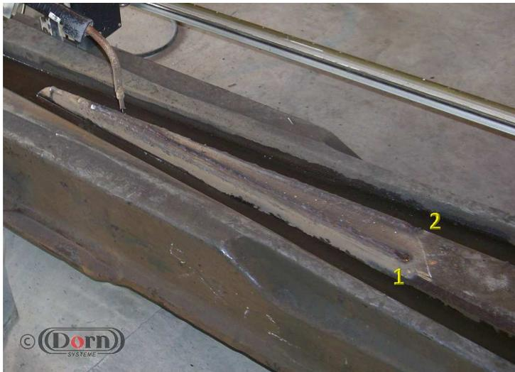
Multi Area welds with automatic count-down timer for “cold” rail.
